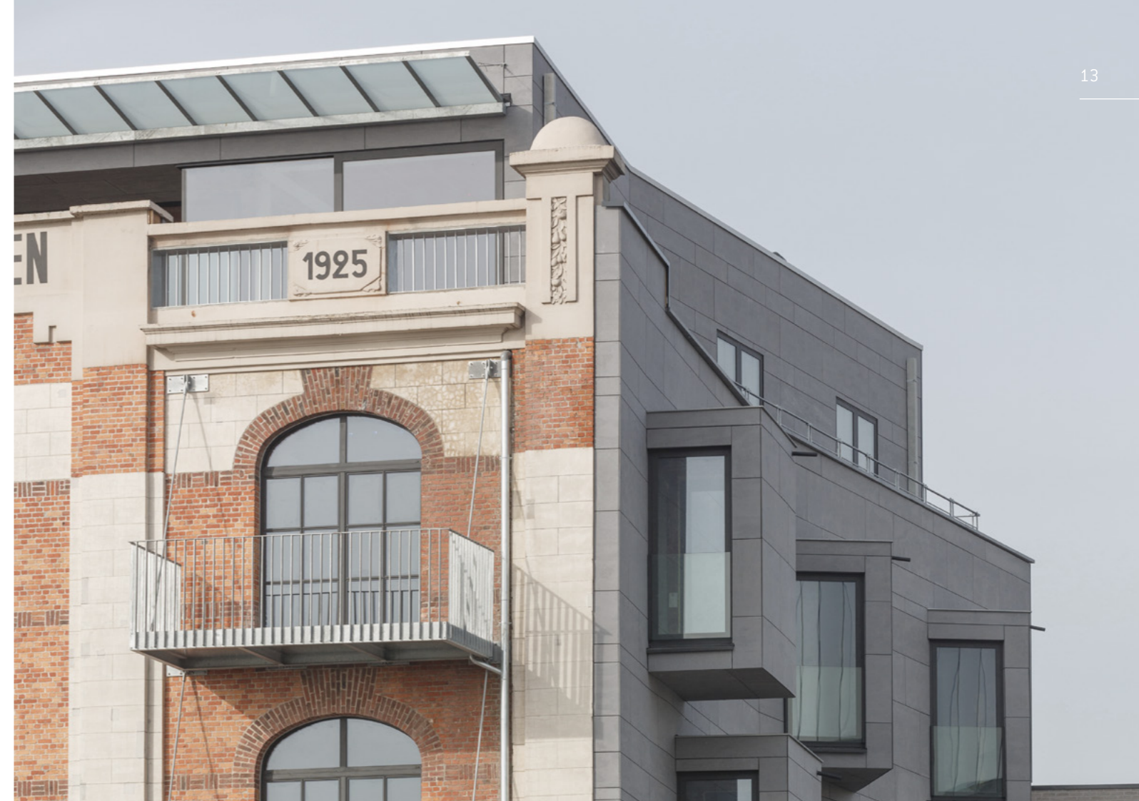
Peynsaert Architecten Aalst, Belgium | EQUITONE [tectiva]®
