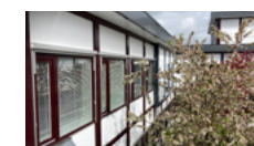
Nij Smellinghe, Drachten, NL Hospital renovation with reused façade panels from 1996
