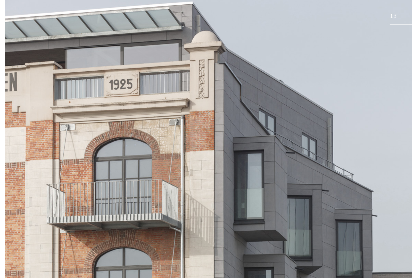
Peynsaert Architecten Aalst, Belgium | EQUITONE [tectiva]®
