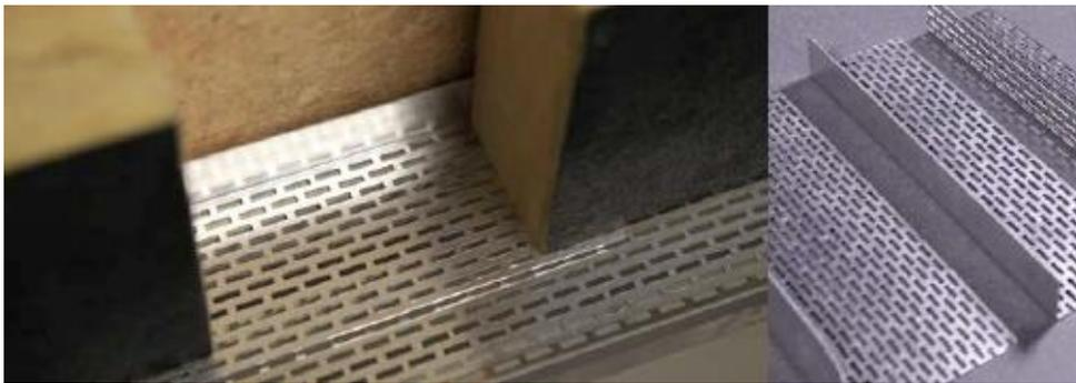
These openings need to be protected against entry of birds and vermin into the cavity space. Failure to protect from these creatures will cause damage to the insulation, cavity space and even the substrate. This is normally achieved by fitting a perforated profile. It is important the perforations are sized correctly to allow air in and out while stopping entry of small creatures.
