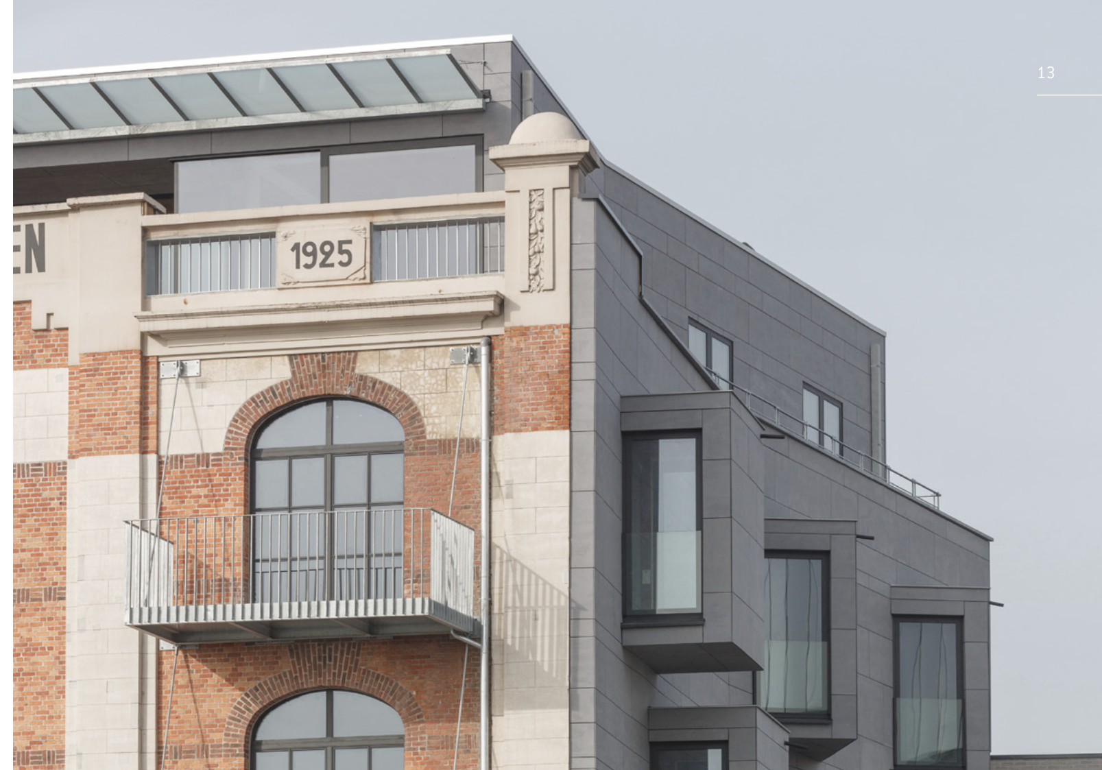
Peynsaert Architecten Aalst, Belgium | EQUITONE [tectiva]®
