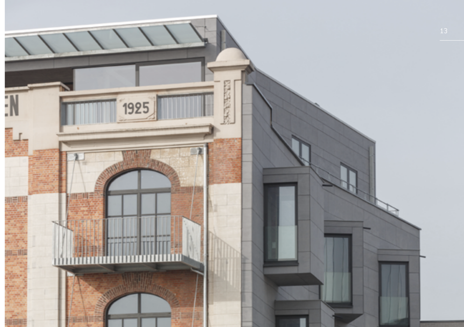
Peynsaert Architecten Aalst, Belgium | EQUITONE [tectiva]®
