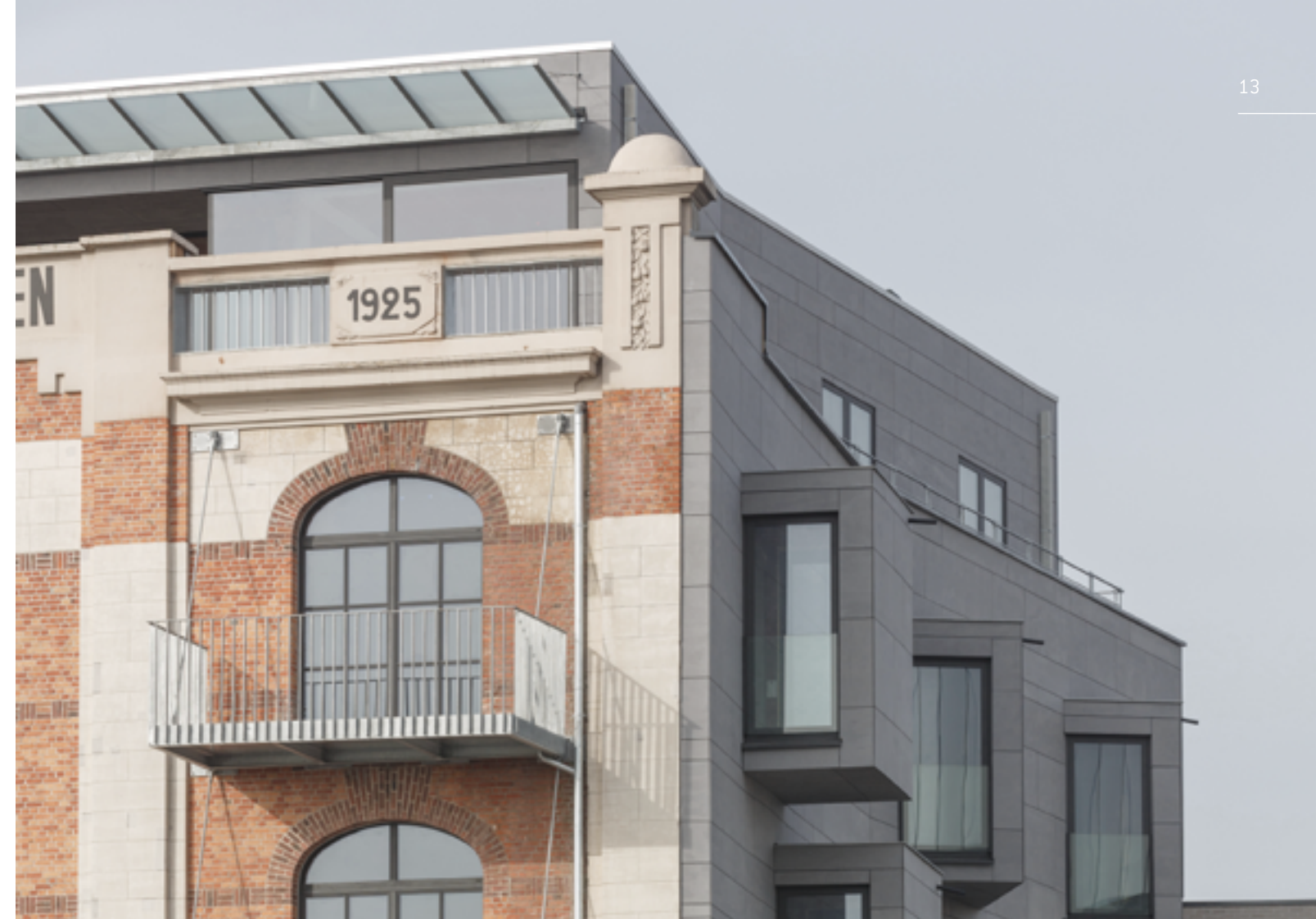
Peynsaert Architecten Aalst, Belgium | EQUITONE [tectiva]®
